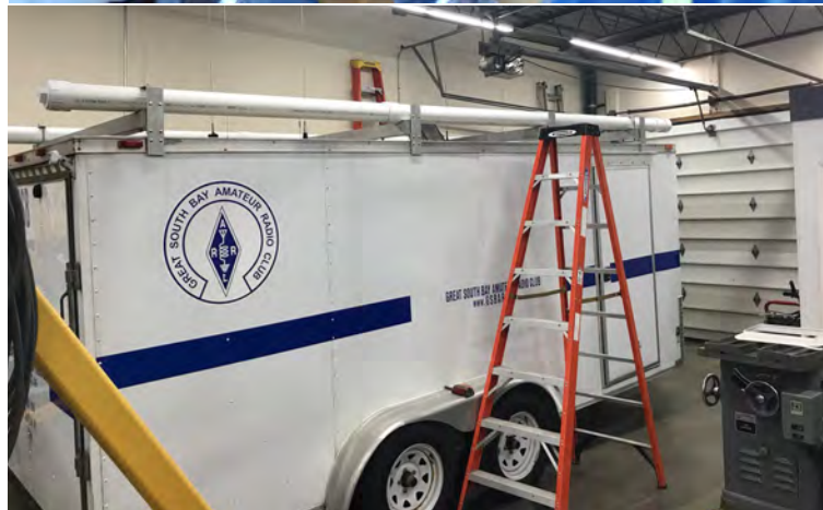
(Top) Installing NUCs and new monitors. (Bottom) Trailer at W2YW’s shop ready for roof-mounted AC installation.
